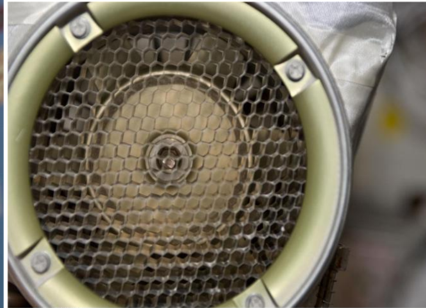
Japanese Pressurized Module Stbd Fwd IMV Fan (Inlet)
